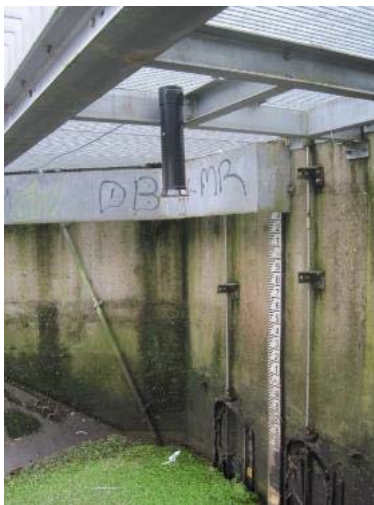
Urban Berkshire Flood alleviation. Provision for GSM/GRPS logger
