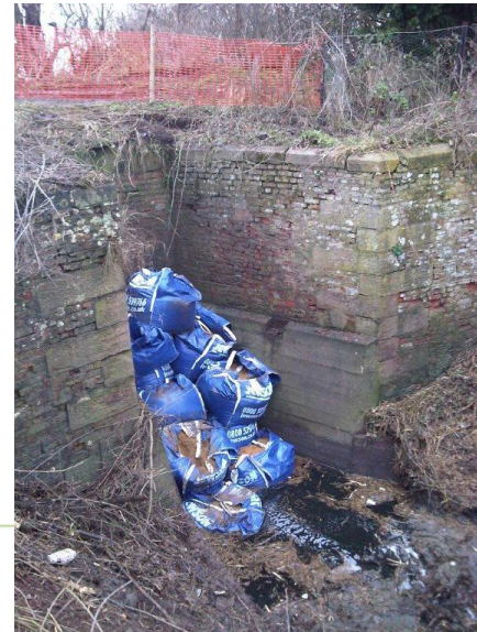
Black Sluice IDB Emergency seal of tidal sluice (Dec 2013)
