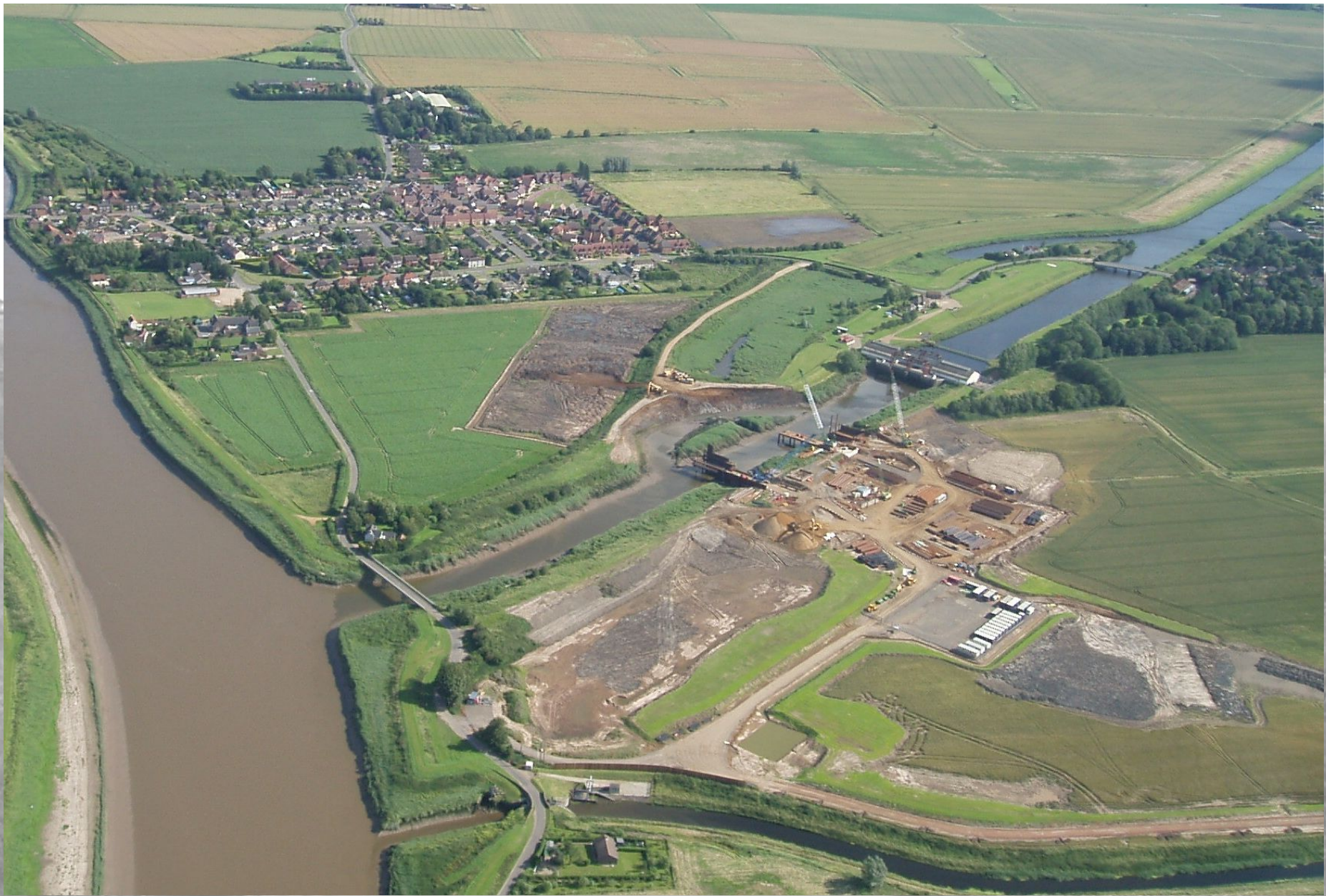
Construction begins on St Germans Pumping Station
