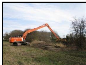
North Level IDB Channel works (part of Nene Washes Scheme)
