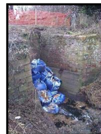
Black Sluice IDB Emergency seal of tidal sluice
