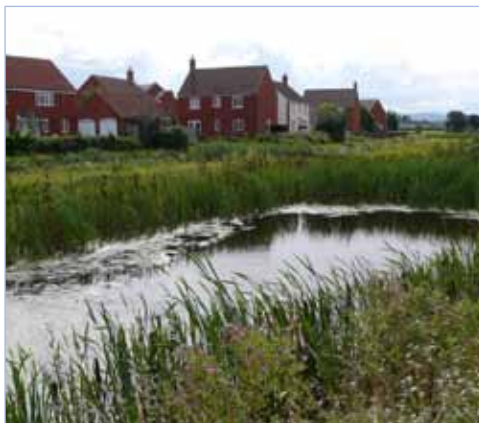
Sustainable Development SuDS for a new housing development in Bridgewater (Source: Phil Brewin)
