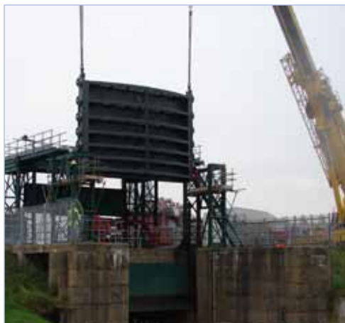
Constructing Sluice Refurbishment; South Holland IDB
