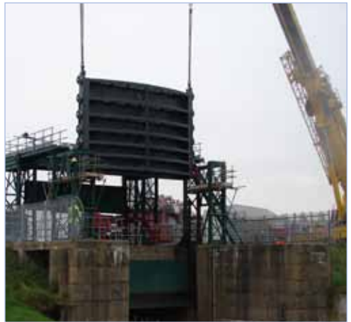
Constructing Sluice Refurbishment; South Holland IDB (Source: Karl Vines)
