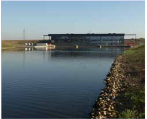
Capital Investment The Middle Level Commissioners' New St. Germans Pumping Station (Source: David Thomas)
