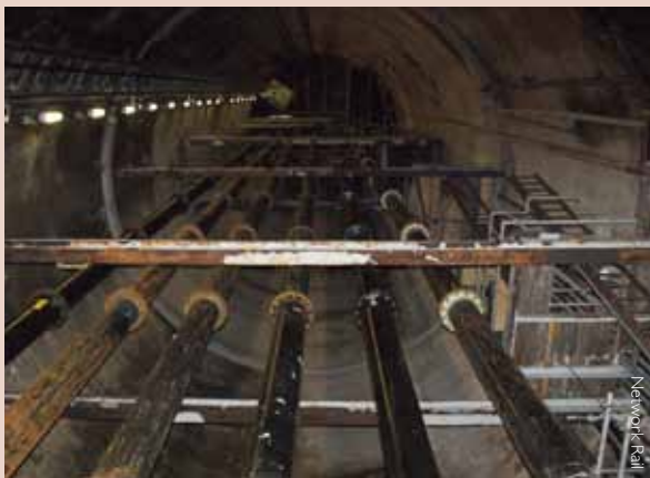
The pumping system in the Severn Tunnel
