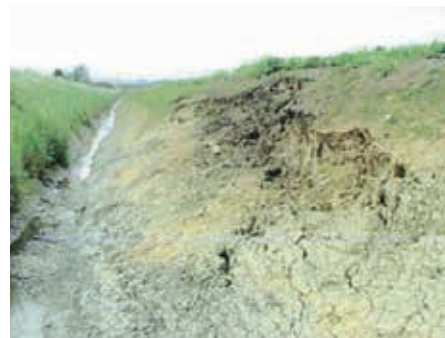
Figure 1 Bank slip caused by a land drain or poor soil structure
