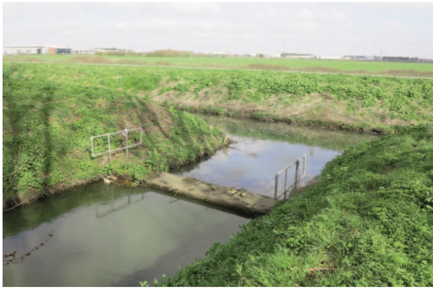
Figure 3 The entrance to the reservoir showing the concrete structure over which water flows in times of high rainfall
