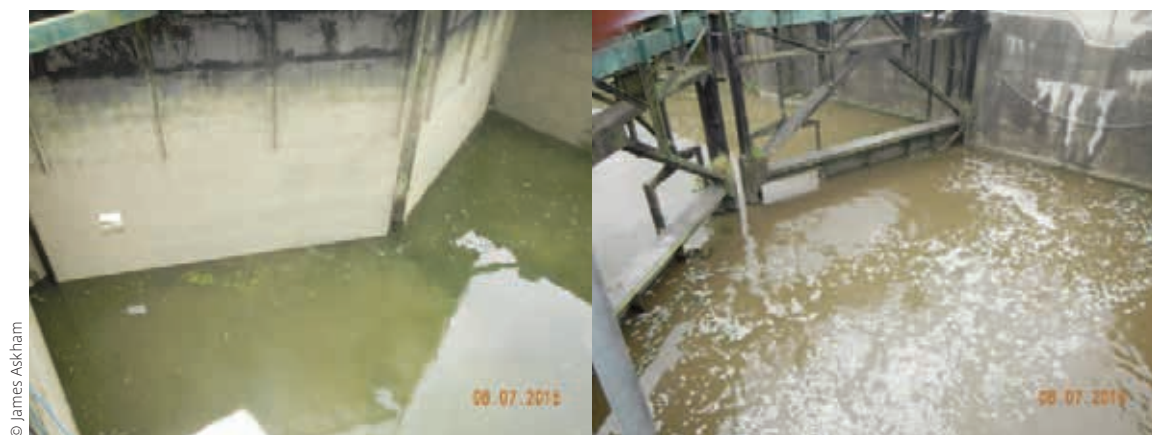
Figure 2 New penstock in outer tidal doors (left) and existing overshoot penstock on internal doors at top of tide (right)
