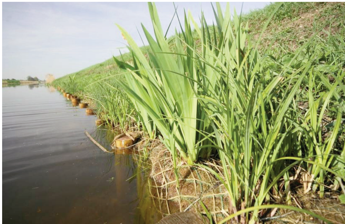
Figure 1 - Coir rolls on the Sixteen Foot River near Bedlam Bridge four months after installation in January 2009. The coir roll is contained in a net of mesh that plant roots and water voles can penetrate. Yellow flag iris and lesser pond sedge are the plants showing good growth in the foreground.
