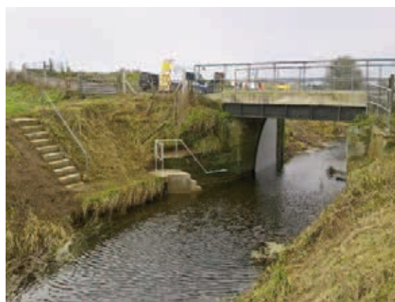
Figure 2 Eldernell sluice with new tilting gate
