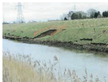
Figure 3 Erosion caused by wave action
