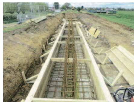
Figure 3 Wave wall construction underway
