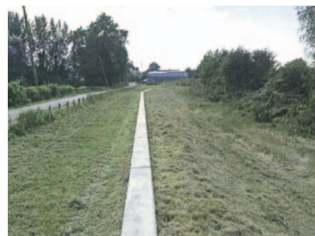
Figure 4 Wave Wall construction completed
