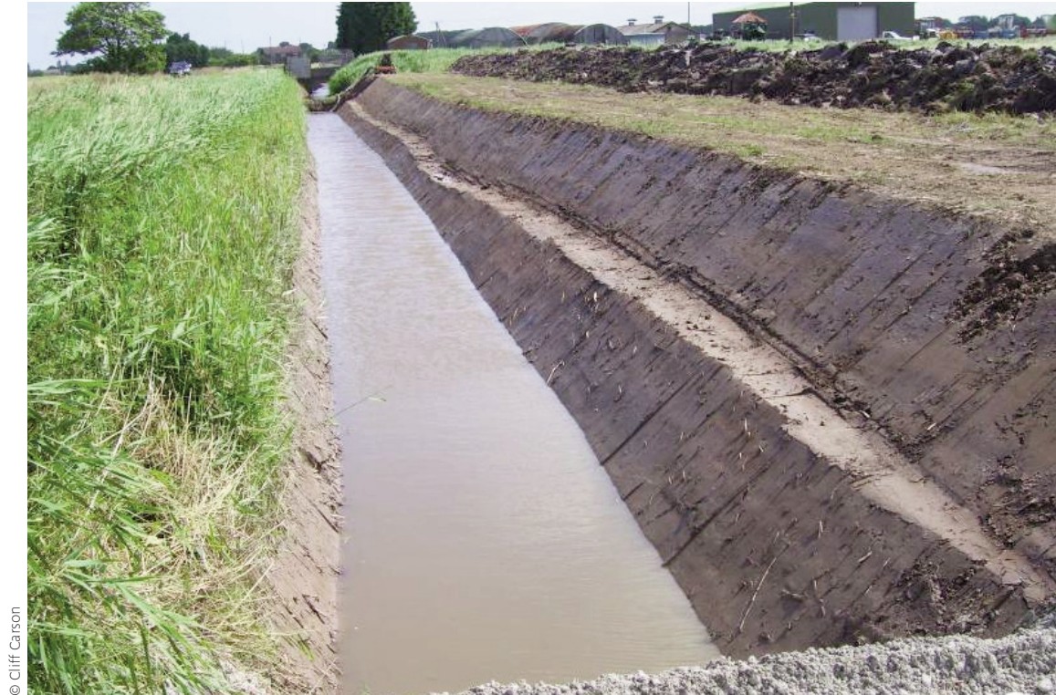
Figure 2 Newly formed berm
