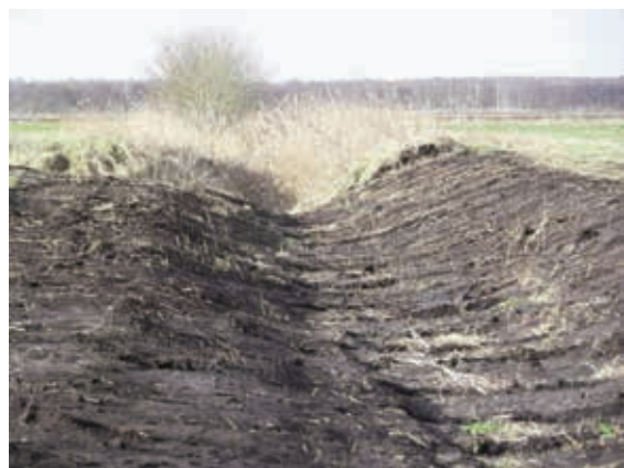
Figure 2 Re-profiled ditch
