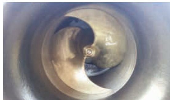
Figure 2 The impeller of one of the new fish friendly pumps installed at the station
