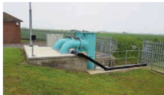
Figure 1 The new fish friendly pumps and eel pass
