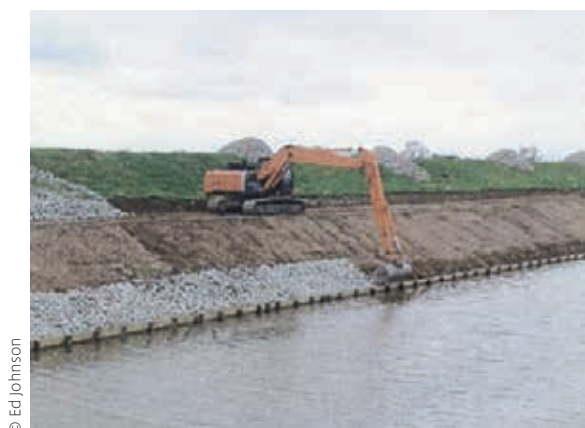
Figure 8 Gabion stones being placed behind timber piles and boards
