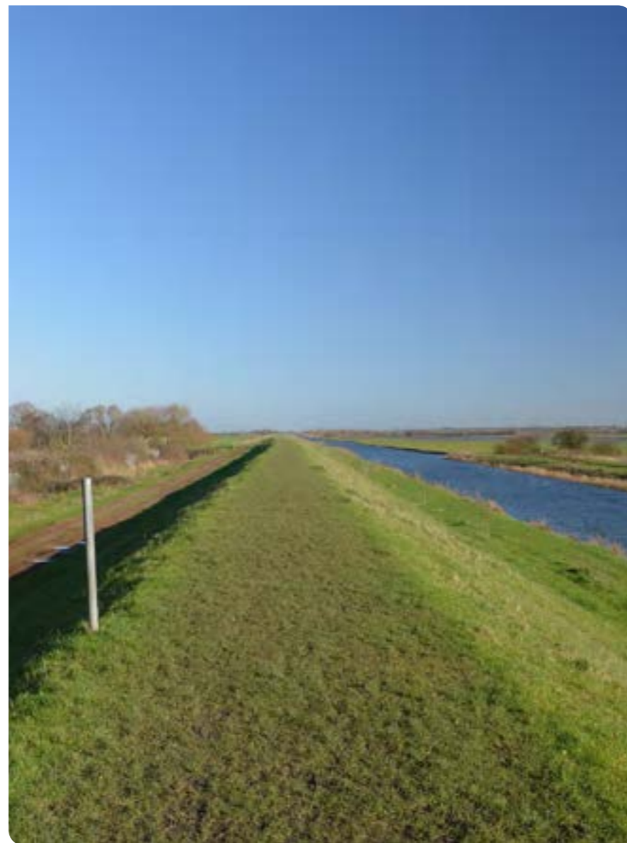
Flood Embankment on the River Delph
