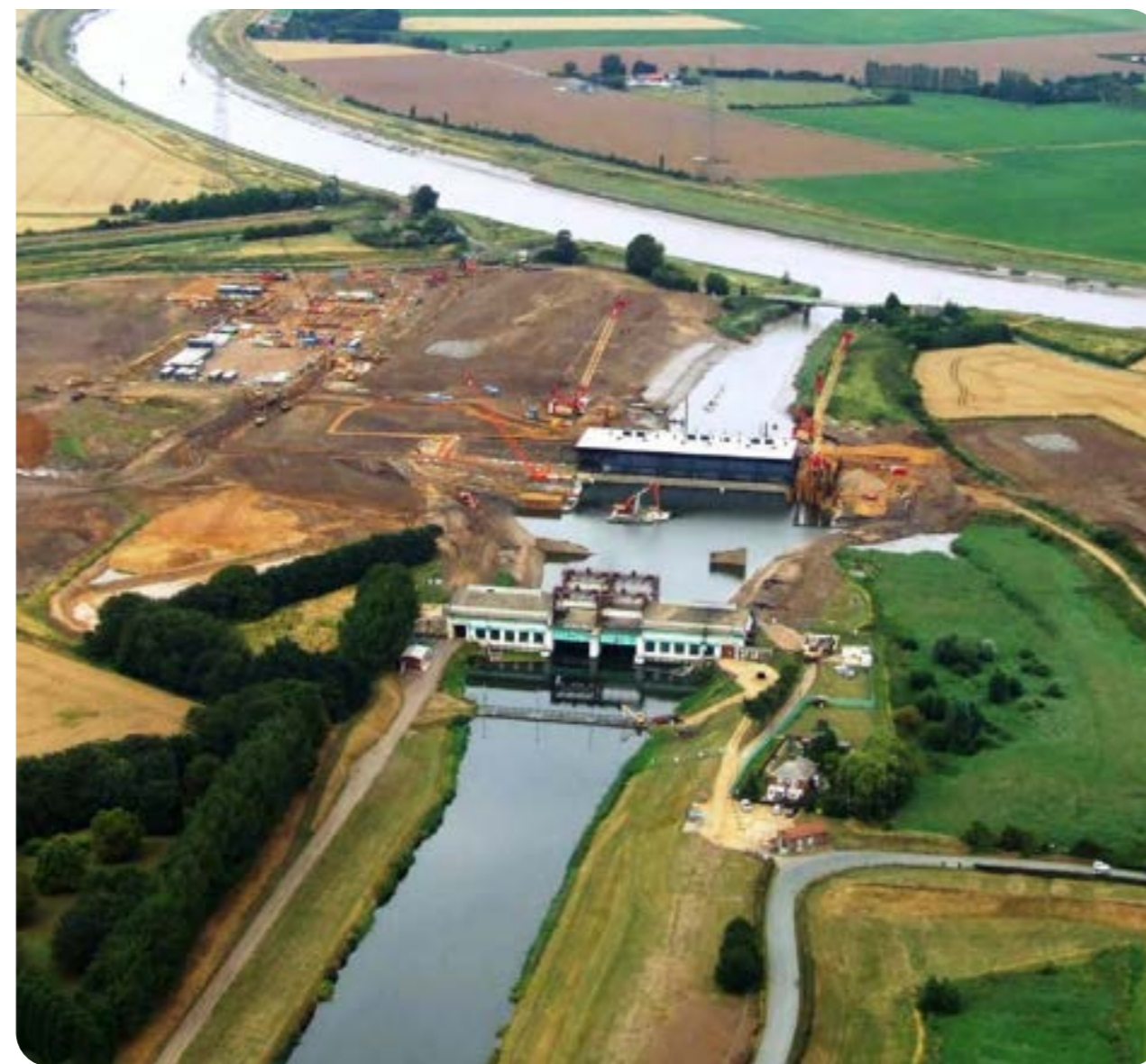
Construction of New St Germans Pumping Station
