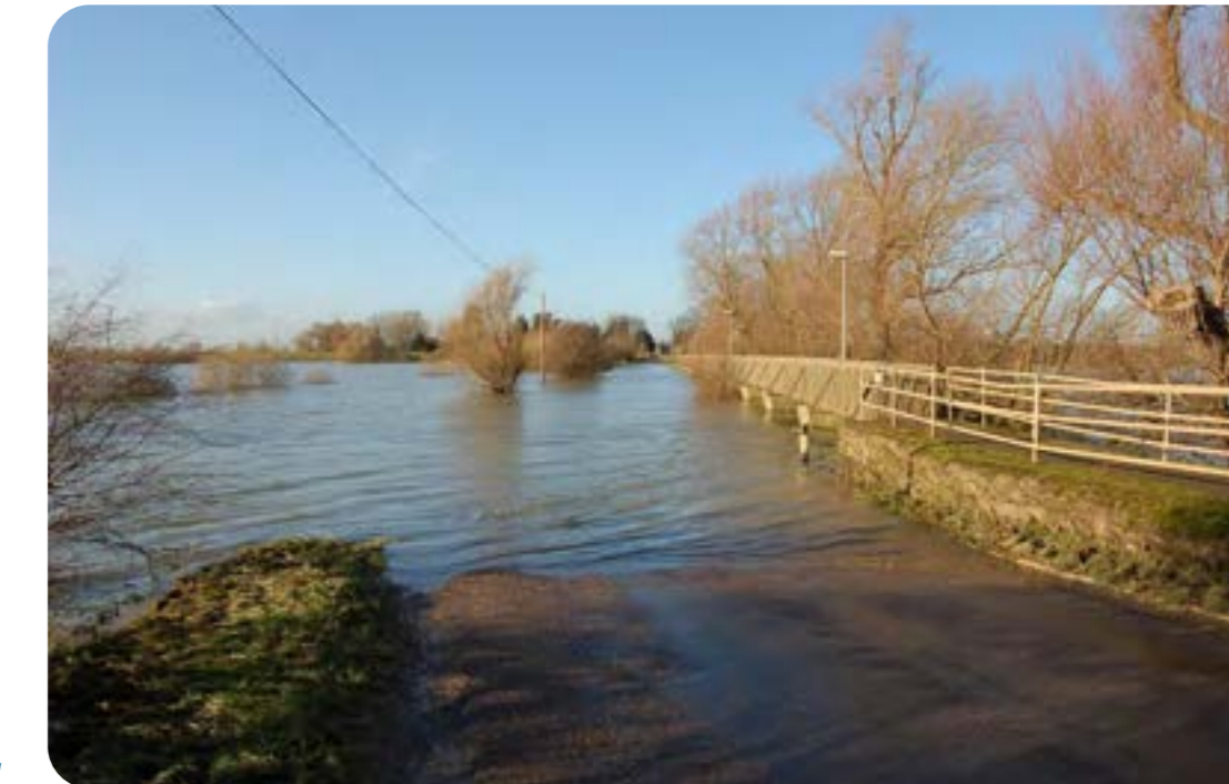
Flooding at Ouse Washes - Sutton Road
