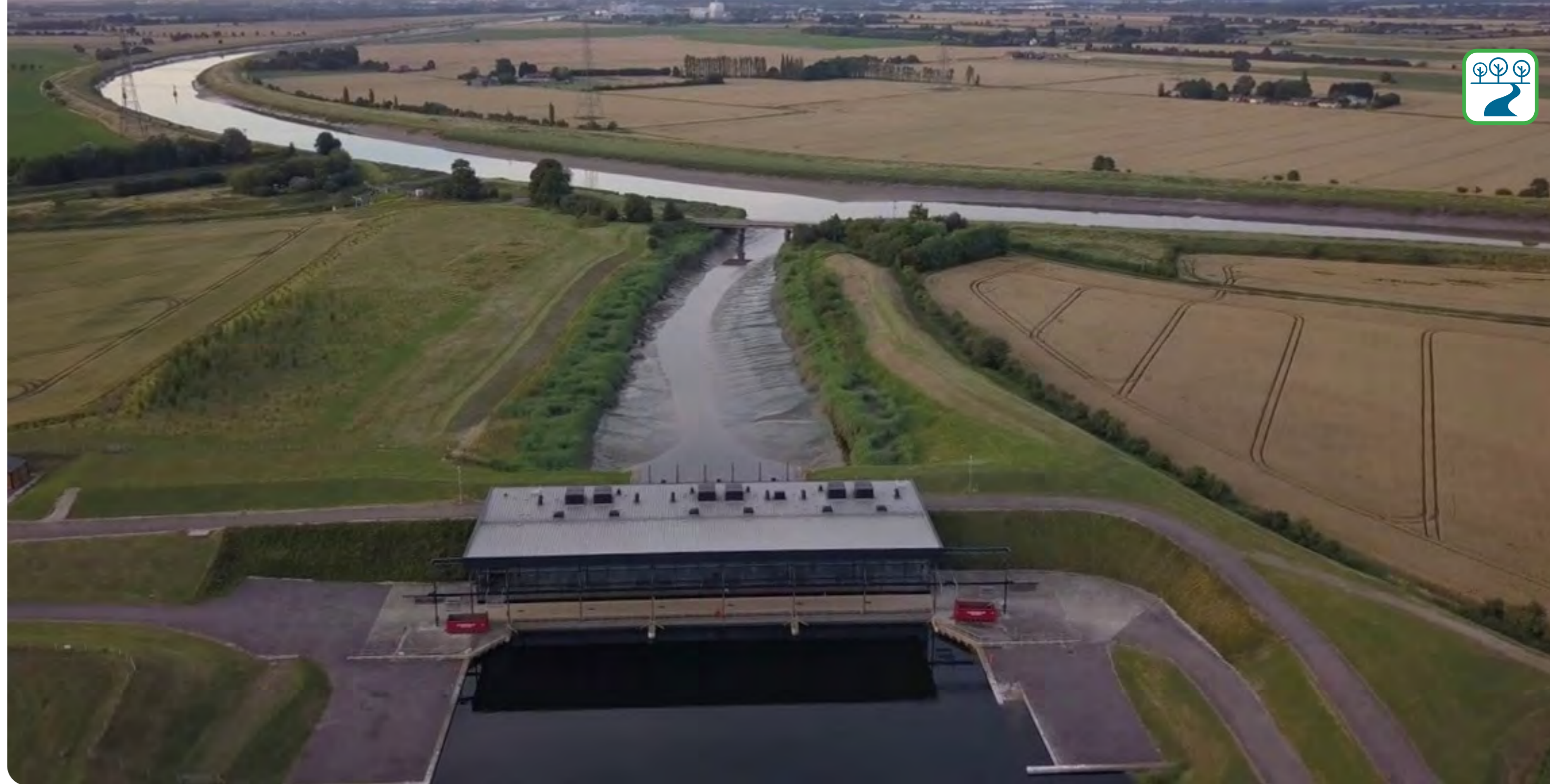
Figure 21: St Germans Pumping Station
