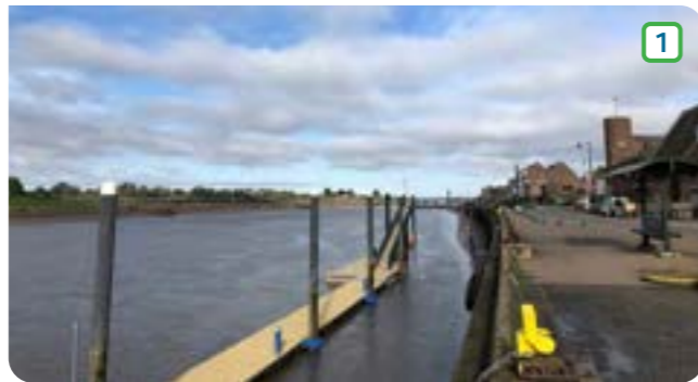
The River Nar flows northwards from the A47 in the King's Lynn area until it reaches Wisbech Road at which point it turns northwest and discharges to the River Great Ouse via a sluice at Hardings Way. For the times when discharge is tide locked, a storage area has been created along part of Blubberhouse Creek through excavation of the area. There is also a diversion channel to the Flood Relief Channel for high flows.
