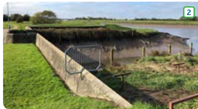
The River Nar flows northwards from the A47 in the King's Lynn area until it reaches Wisbech Road at which point it turns northwest and discharges to the River Great Ouse via a sluice at Hardings Way. For the times when discharge is tide locked, a storage area has been created along part of Blubberhouse Creek through excavation of the area. There is also a diversion channel to the Flood Relief Channel for high flows.
