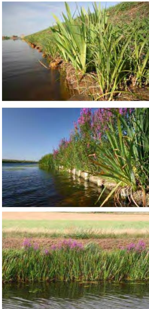
Figure 1: Examples of coir rolls installed on banks
