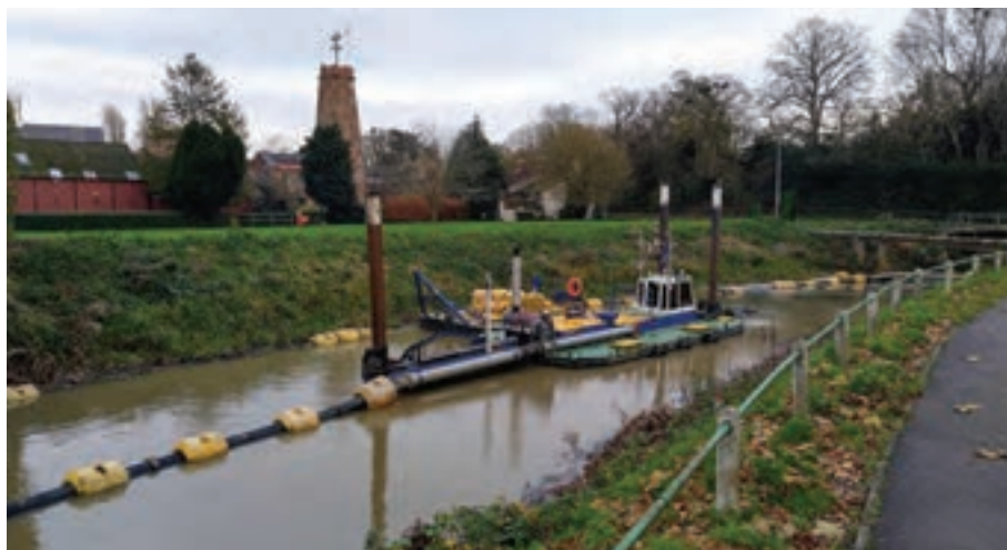
A cutter suction dredger in Wainfleet All Saints
