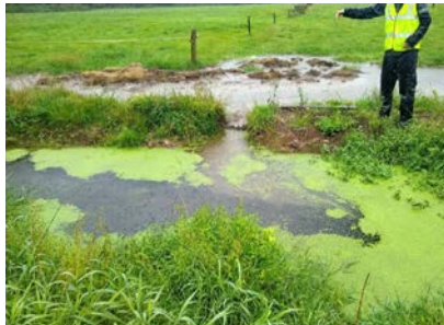
Excavation in a farmers drainage ditch
