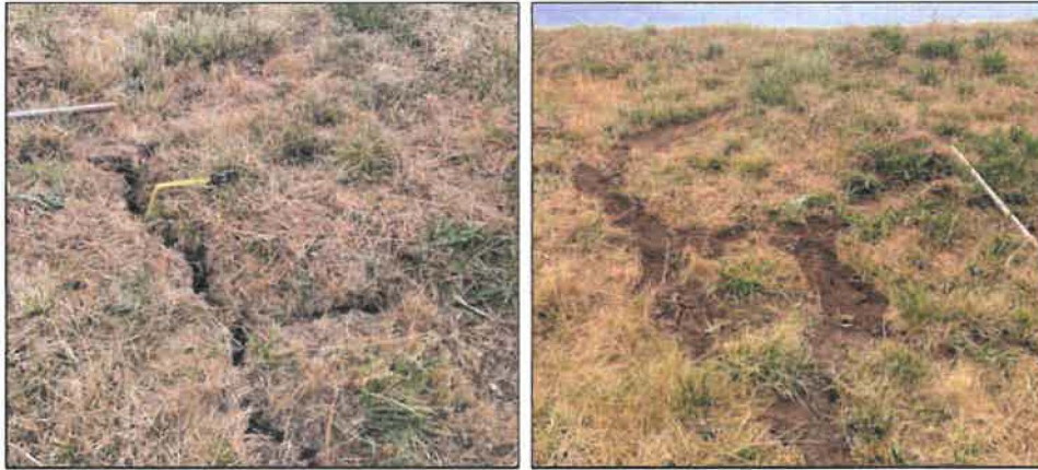
Photo 6 & 7: Donna Nook bank repairs to ensure stability with the forecast rain
