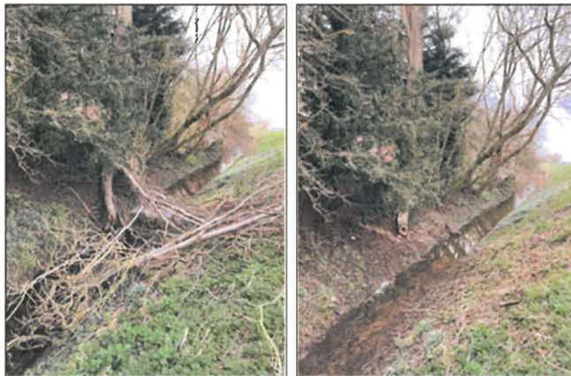
Photo 17: Removal of fallen tree on Carr Dyke near Billingham
