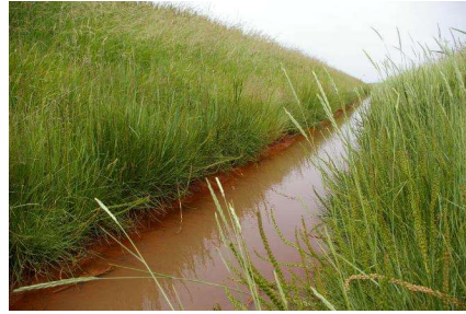
Drains behind sea banks
