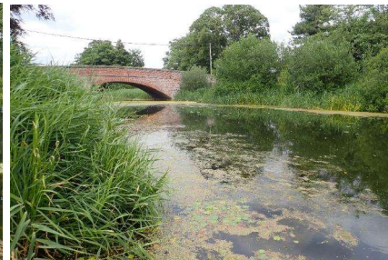
Maud Foster Drain (Rawson's Bridge)
