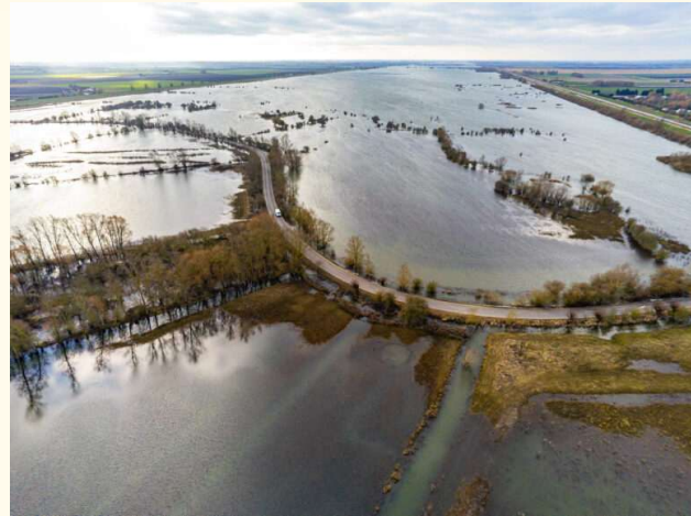
Source: EA - Views of the flooding surrounding the A1101 at Welney.
